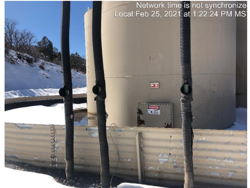
Photo #2987 Flow line heating insulation open ended and not capped.
