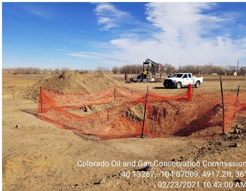
Photo 1 – Remediation area; fencing around open excavation beginning to fall
