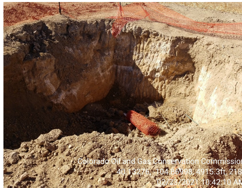
Photo 2 – Remediation area; fencing around open excavation beginning to fall.
