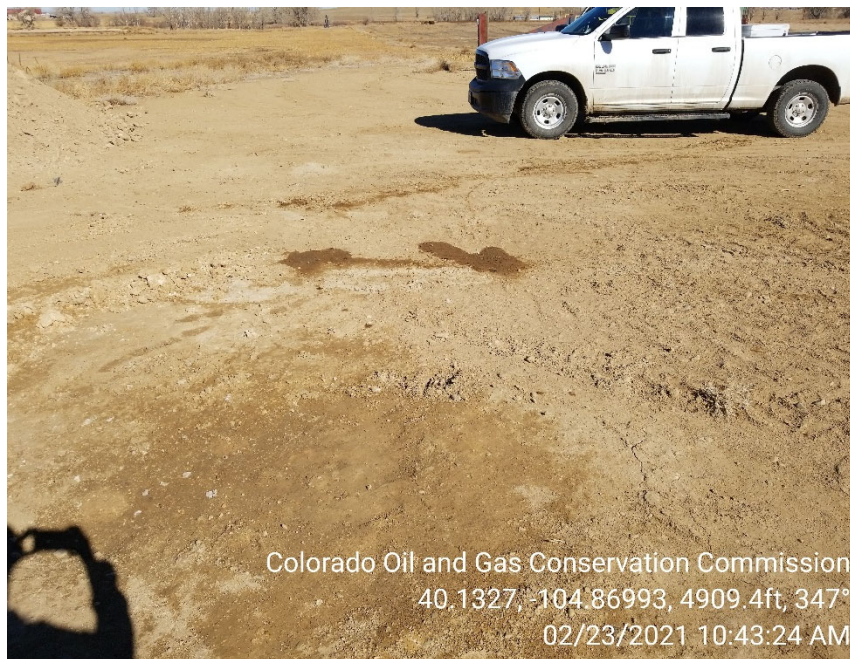
Photo 5 – Surface staining visible outside of excavation area
