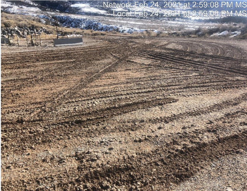
Photo #2976 Rutting present on location due to lack of stabilization.
