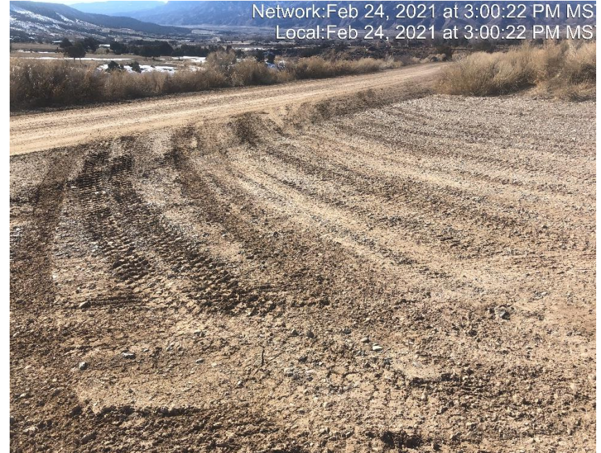
Photo #2979 No form of tracking control at the entrance to location.
