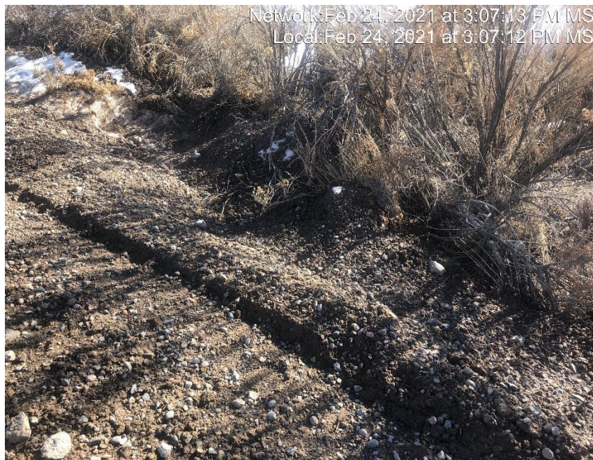
Photo #2982 Sediment has been plowed into ditch and is choking off vegetation.
