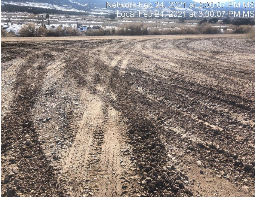
Photo #2978 No form of tracking control at the entrance to location.
