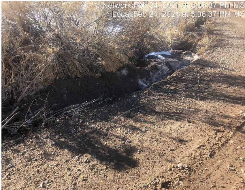
Photo #2980 Sediment has been plowed into ditch and is choking off vegetation.
