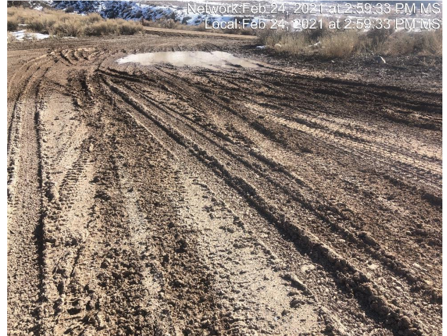
Photo #2977 Rutting present on location due to lack of stabilization.
