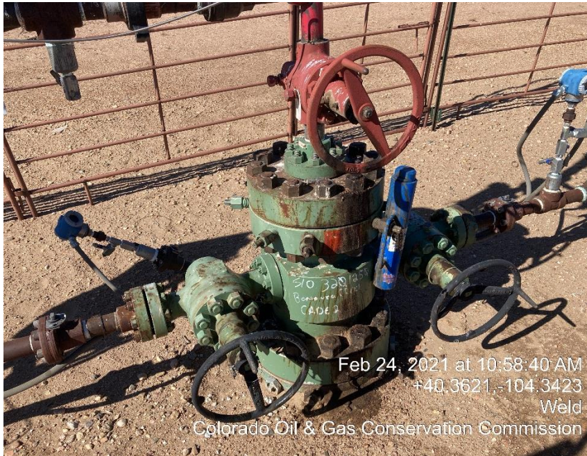
Photo #4 Stained Soil/ Leaking master valve
