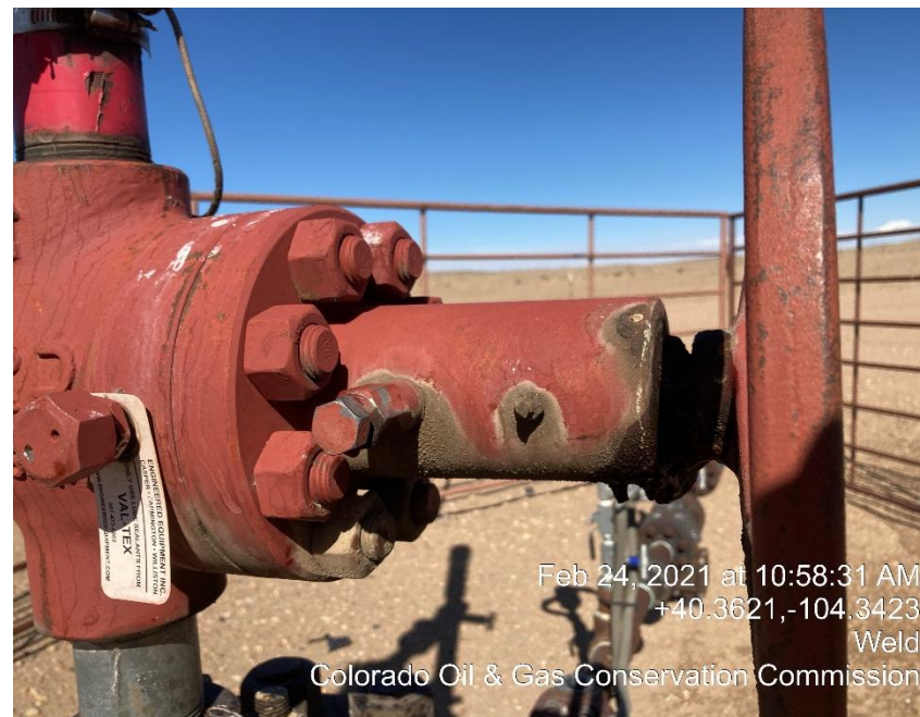
Photo #3 Leaking Master valve
