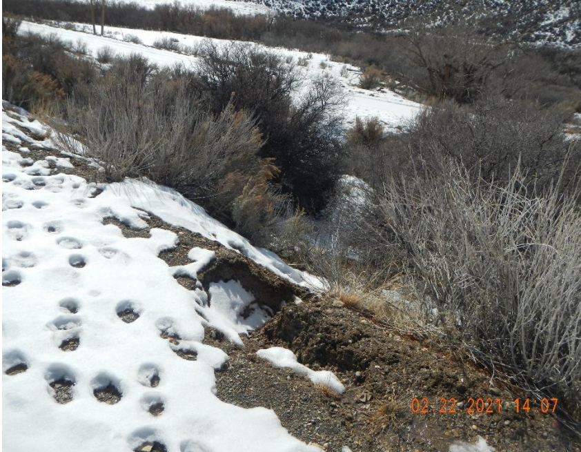
Erosion wash on shoulder of access road up to location.
