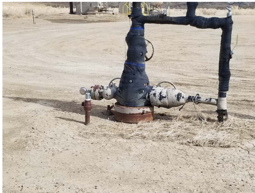
Photo 2. No bradenhead access apparent.
