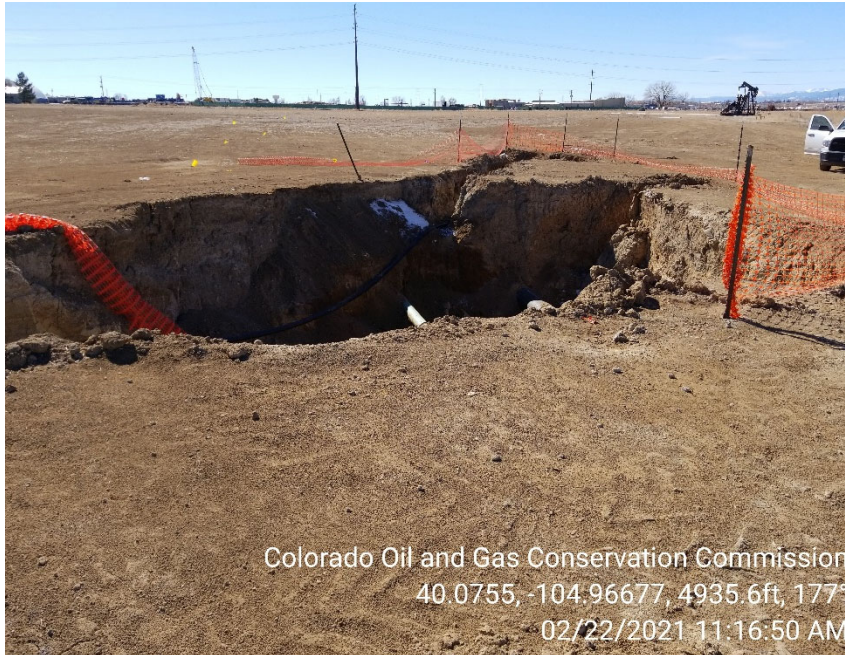
Photo 1 – Spill excavation area. Fencing is down around open excavation.
