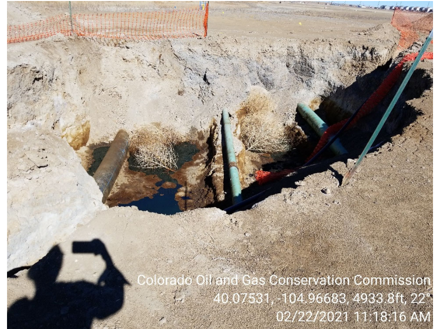
Photo 4 – Free product present in open excavation.
