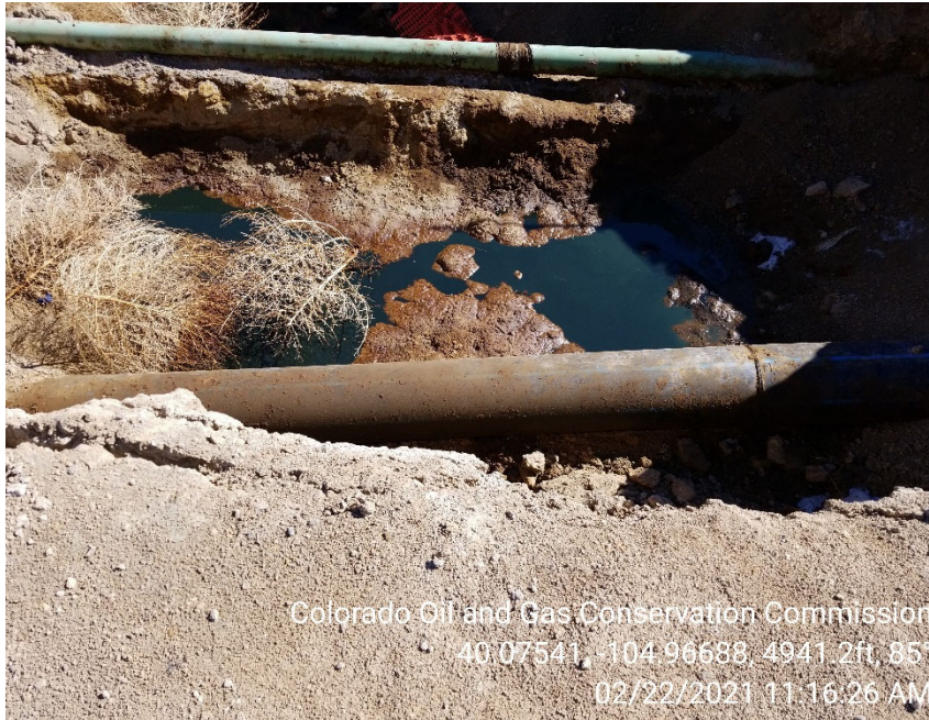
Photo 3 – Free product present in open excavation.
