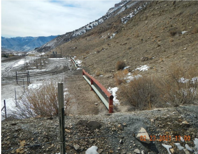
Sediment build up behind falling rock guard rails.
