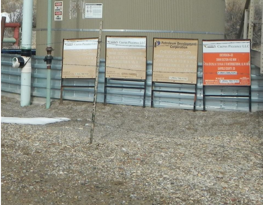
Battery sign missing Operator name.
