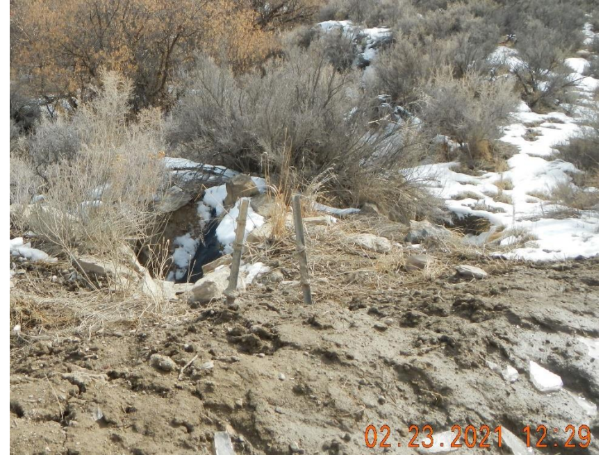
N39.55348 W-108.11985 Erosion damage from culvert outlet.
