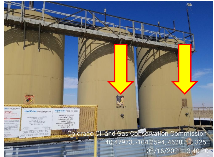
Photo 6 – Signs have faded on Tanks
