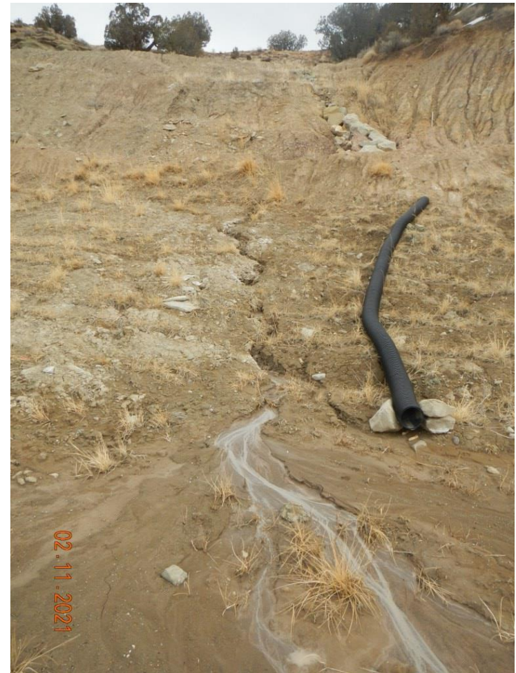
Photo#7: Bypassing/undercutting of BMP on South Cut.
