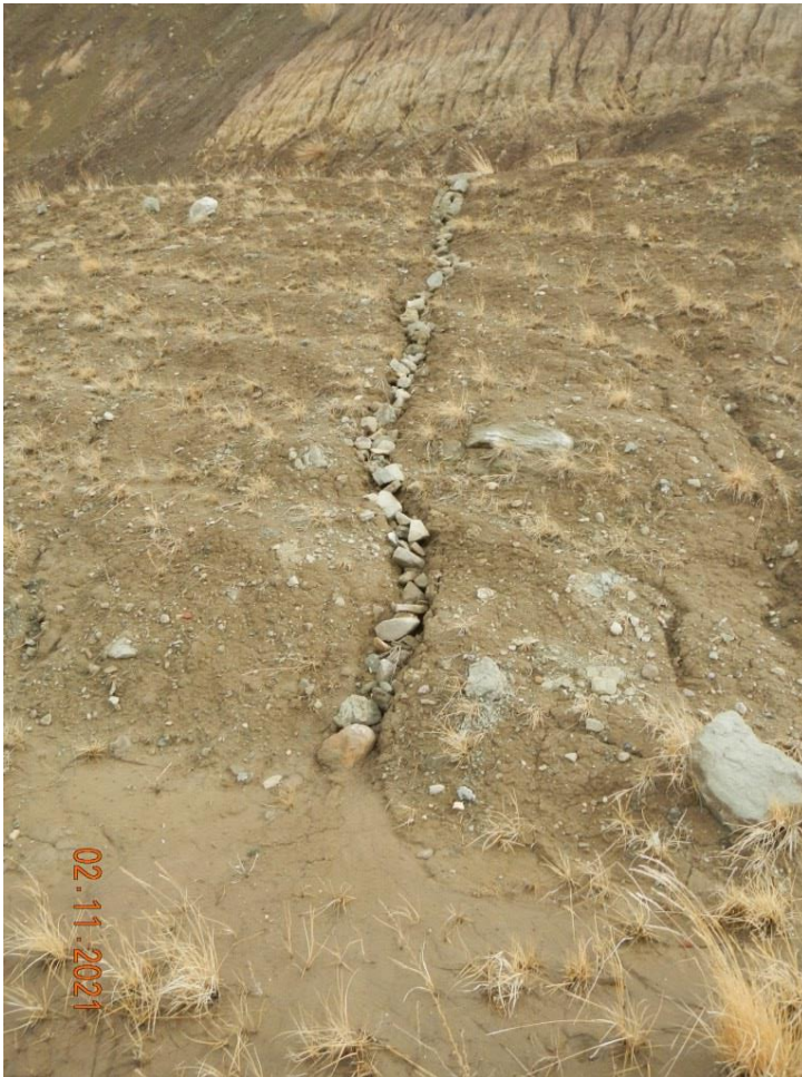
Photo#6: Undercutting of BMP on South Cut.
