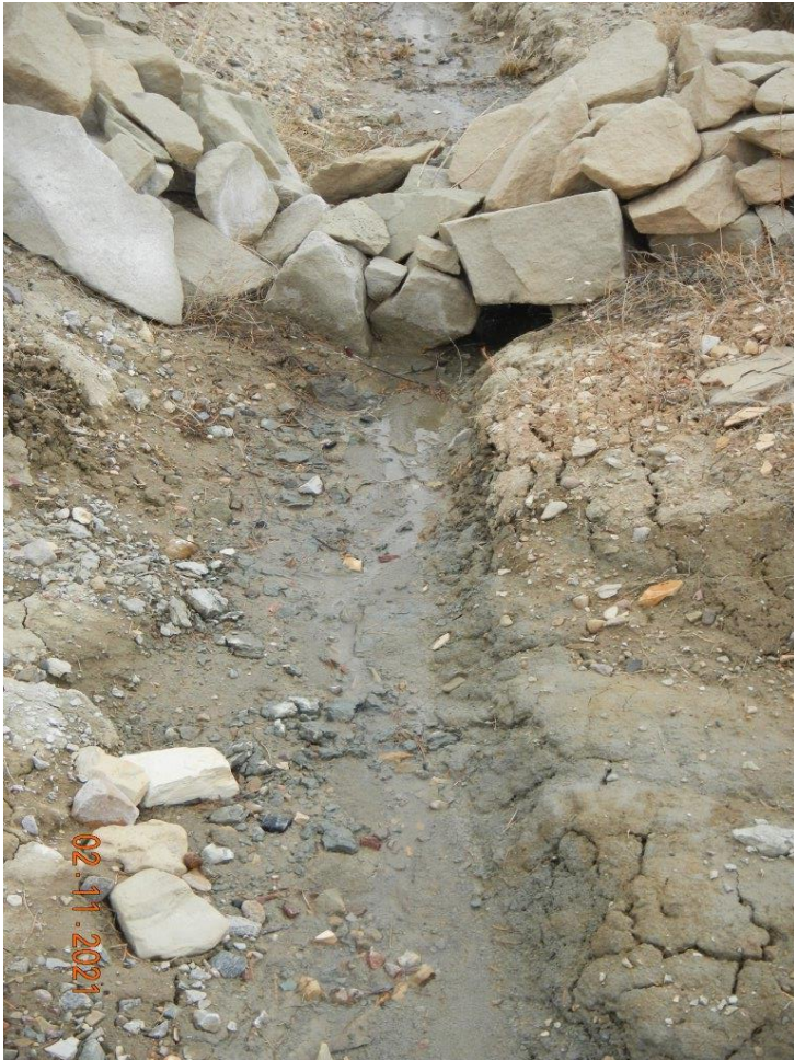
Photo#4: Undercutting of BMP on south Cut.
