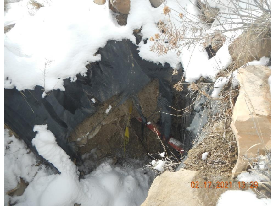
Erosion has exposed pipe line.
