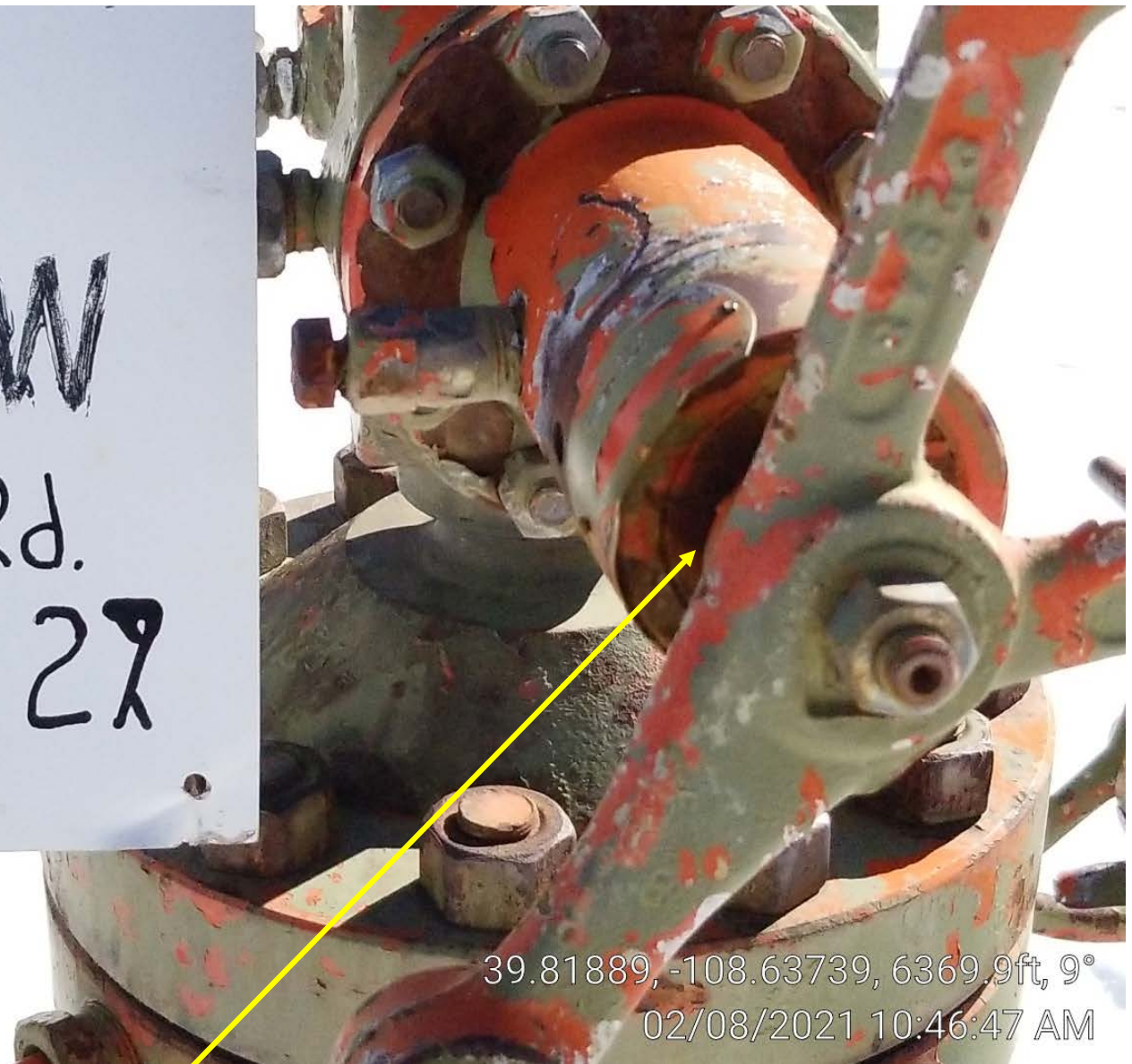
Photo 2. Well gas leak.
