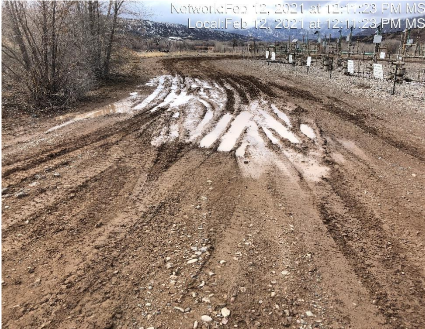
Photo #2900 Rutting present on location due to lack of stabilization.
