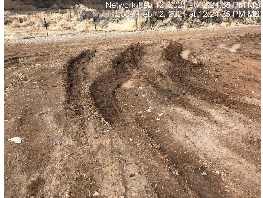
Photo #2901 Rutting present on location due to lack of stabilization.
