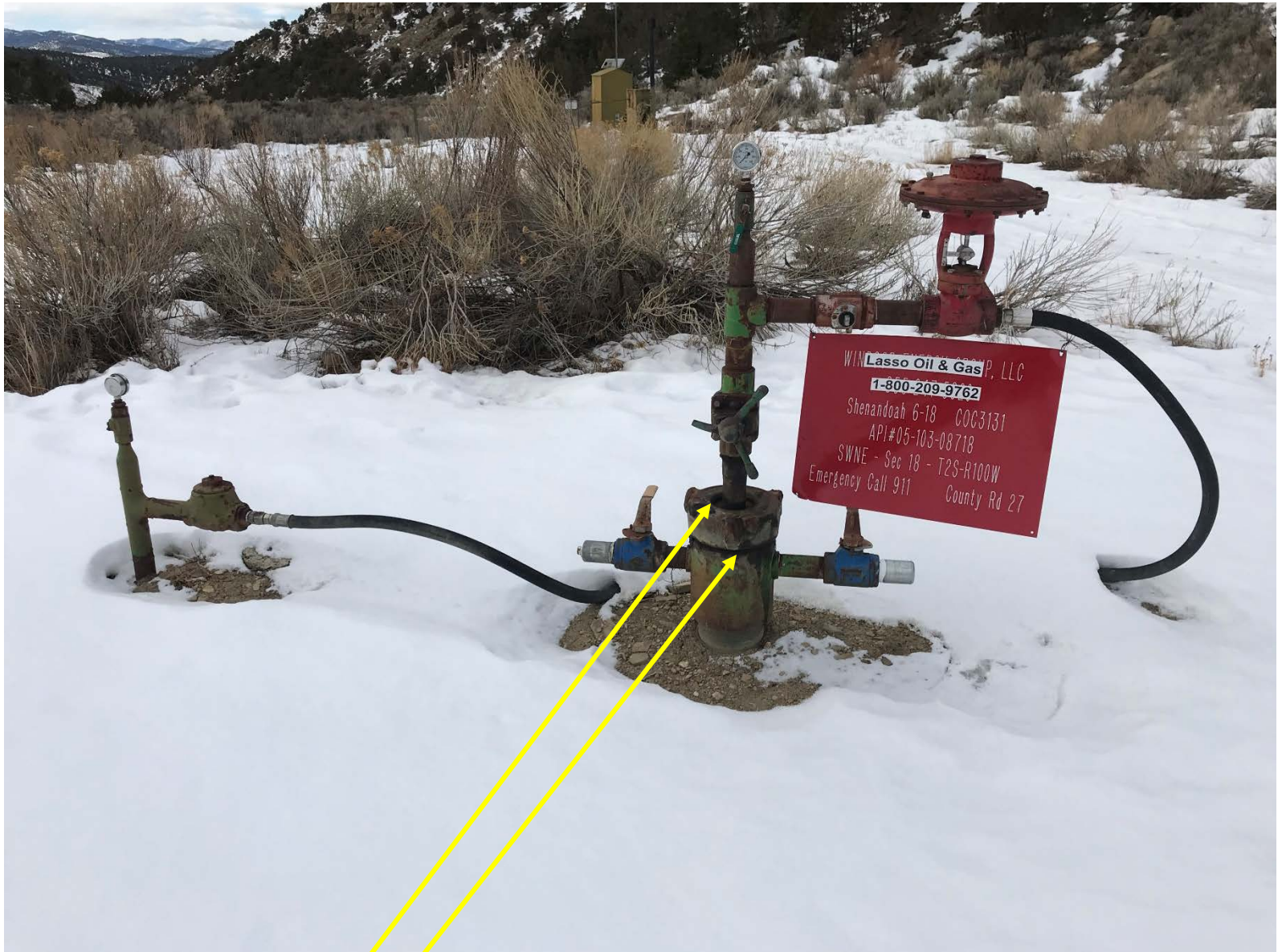
Photo 2. Well gas leaks.
