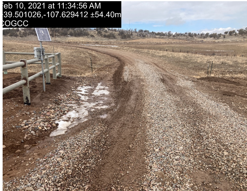
Lack of stabilization/ Lack of tracking controls from follow up inspection
