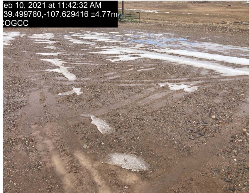
Lack of stabilization from follow up inspection
