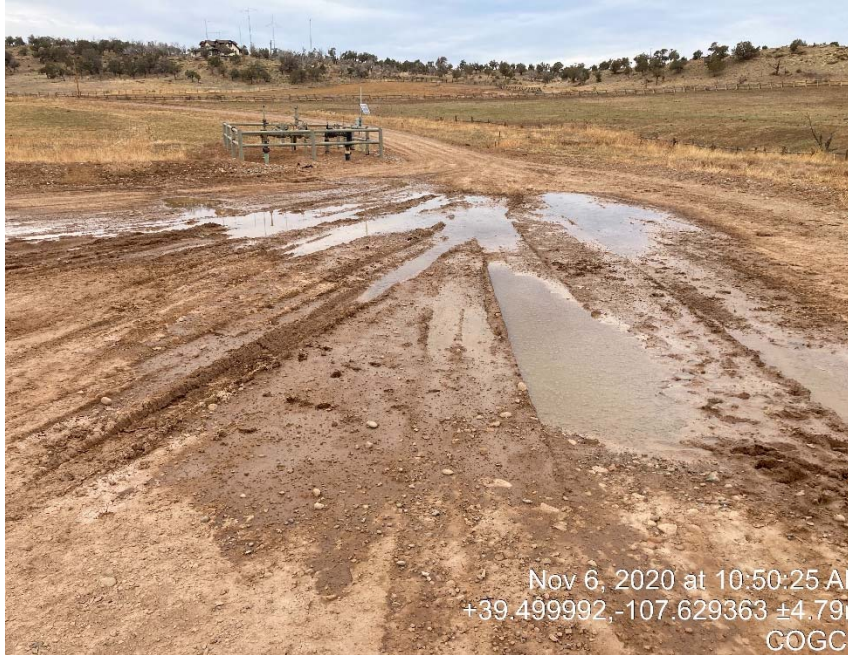
Lack of stabilization from previous inspection
