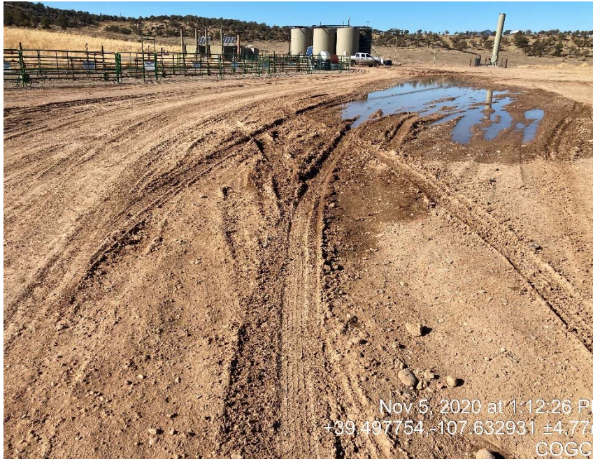
Lack of stabilization from previous inspection
