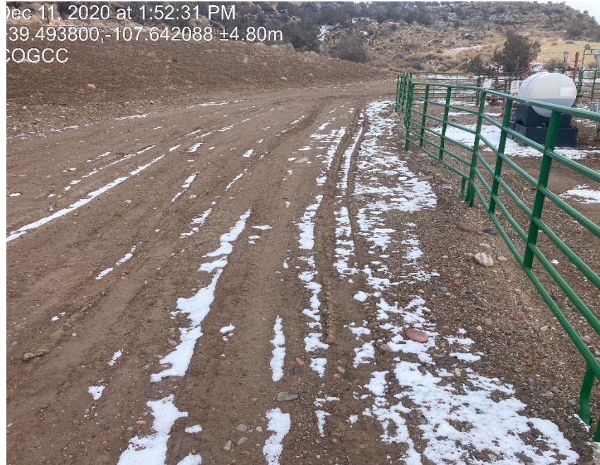
Previous inspection photo of lack of stabilization
