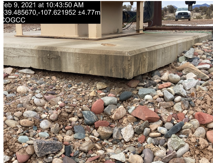
Sediment migration/erosion under combustor (photo from follow up inspection)
