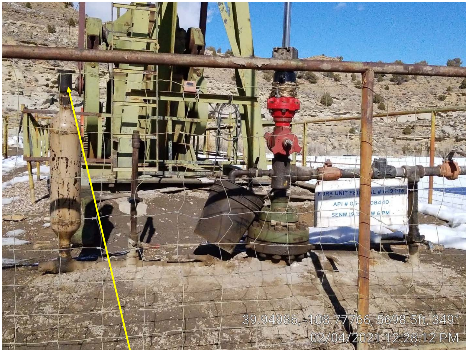
Photo 2. Well gas leak.
