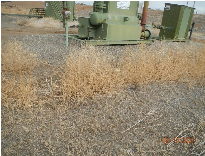
Combustible material (dead/dry weeds) within 25 feet of fired equipment
