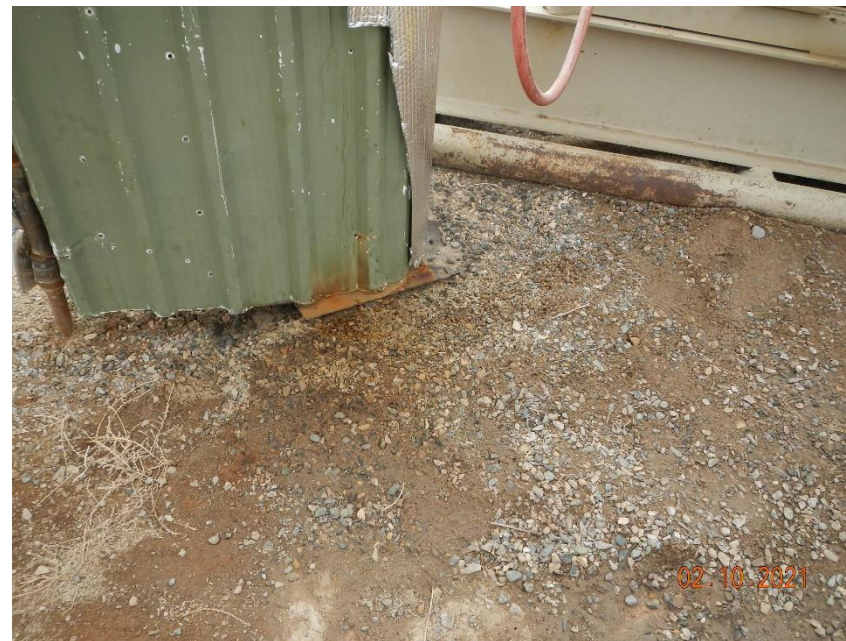
Oil leak/exhaust staining
