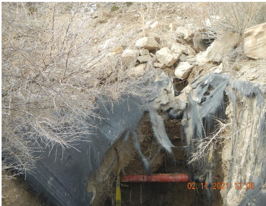
N39.55348 W-108.11985 Erosion damage from culvert outlet.
