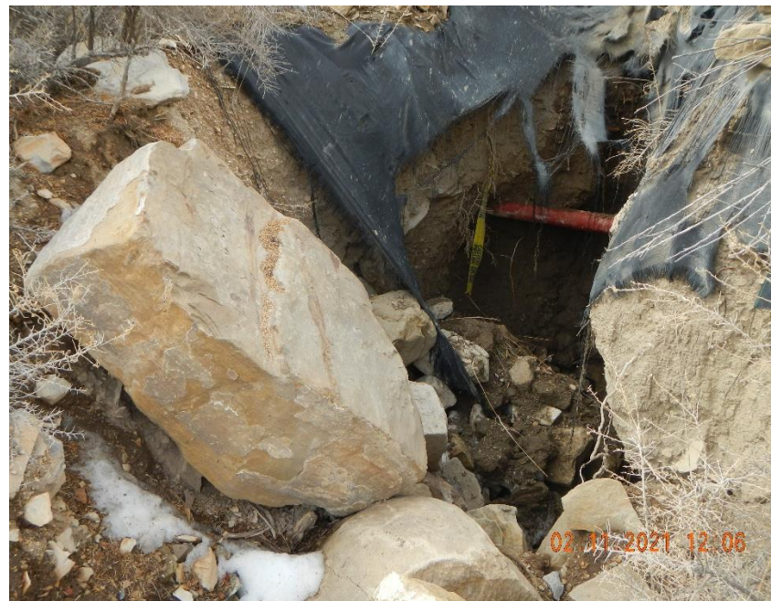
Erosion has exposed pipe line.
