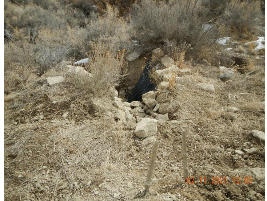
N39.55348 W-108.11985 Sediment build up in culvert outlet. Erosion damage from culvert outlet
