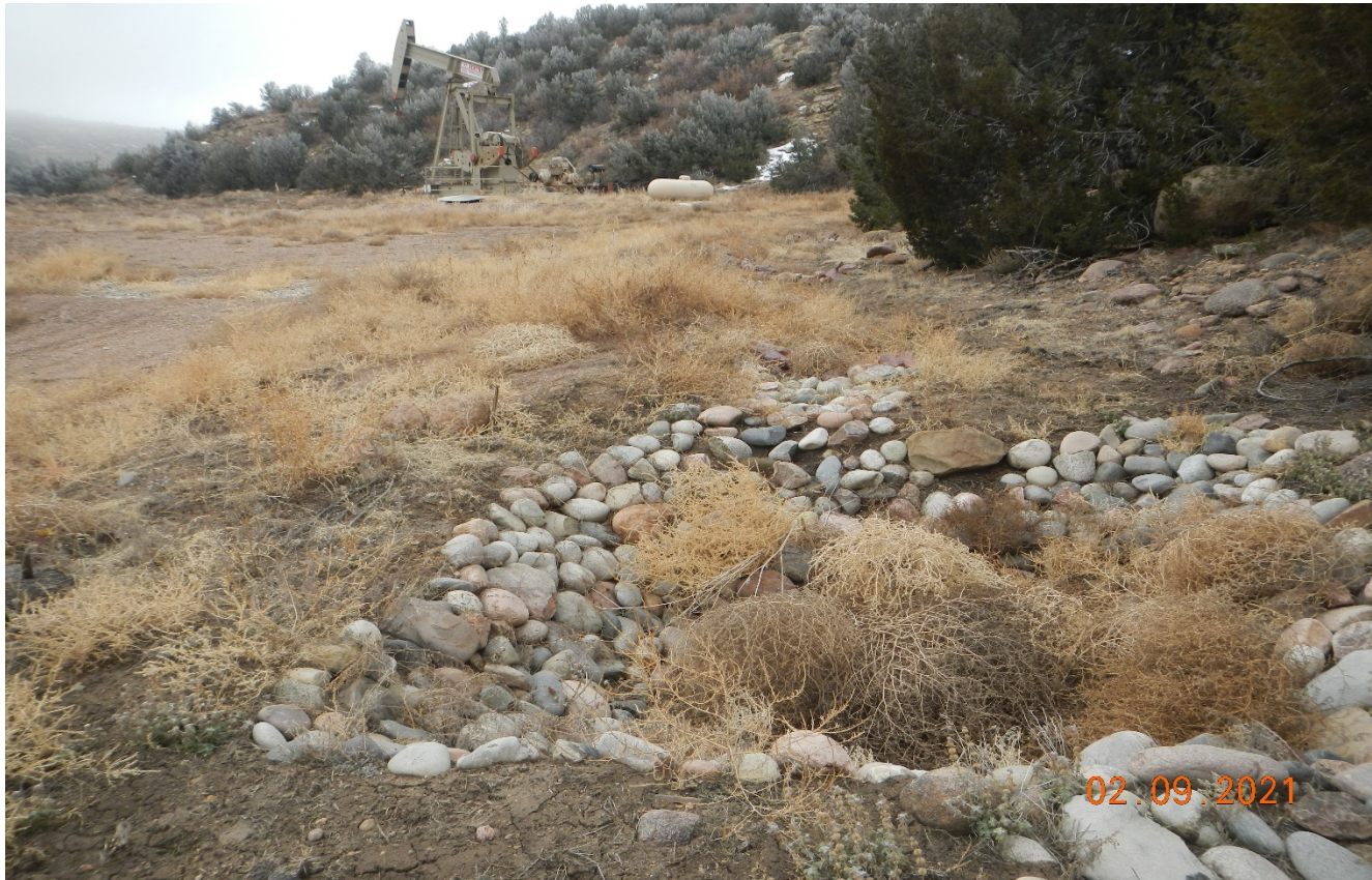
Photo 8. Facing toward the sediment trap. Undesirable weed debris needs to be removed out of sediment trap.
