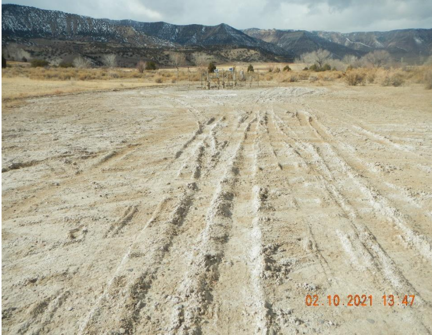
Location shows signs of lack of stabilization BMP's in some areas (rutting is present).
