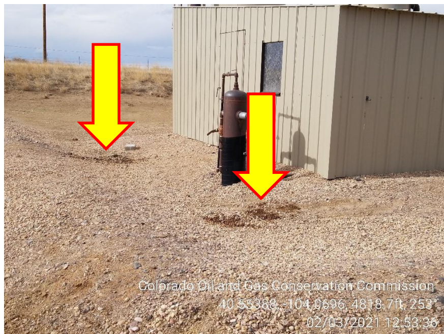
Photo 13 – Heater Treater Shed – Stained Soil
