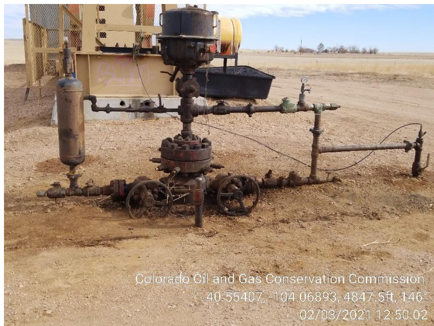
Photo 3 – Wellhead – Stained Soil
