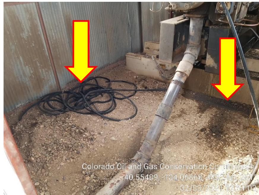
Photo 6 – Gas Engine – Stained Soil – Unused Belts
