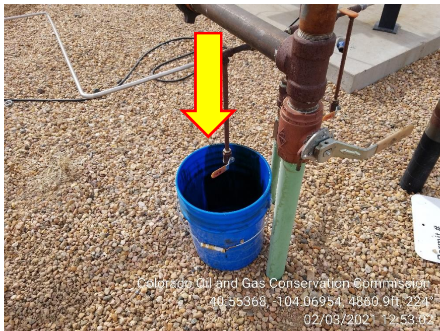
Photo 11 – Oily Waste and no Wildlife Covering at Flare
