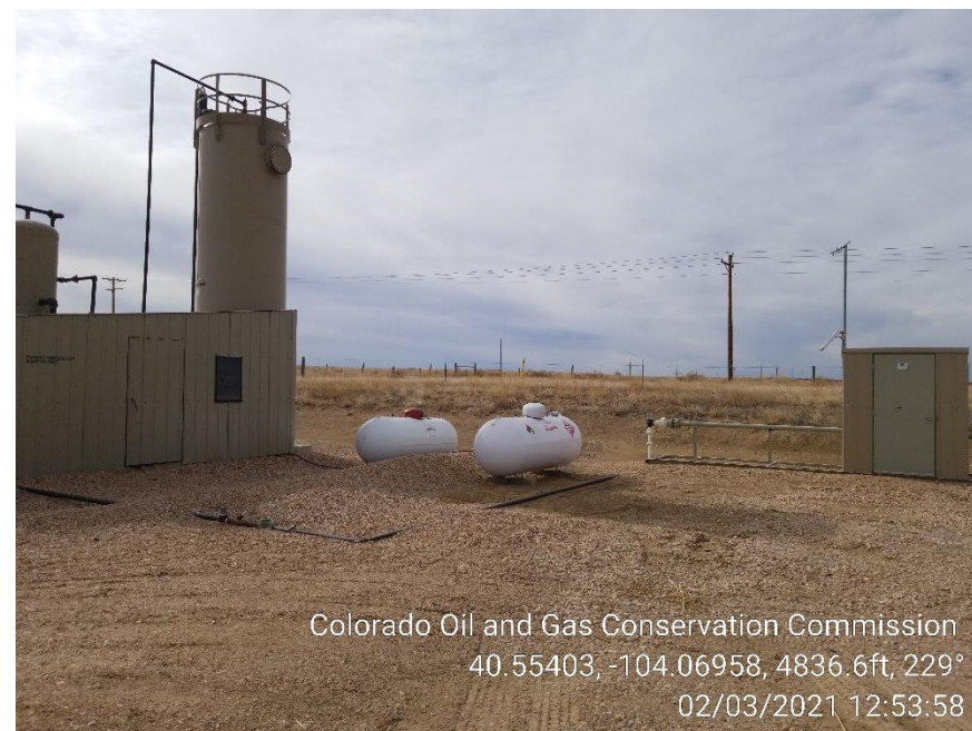
Photo 14 – Heater Treater and Gas Meter
