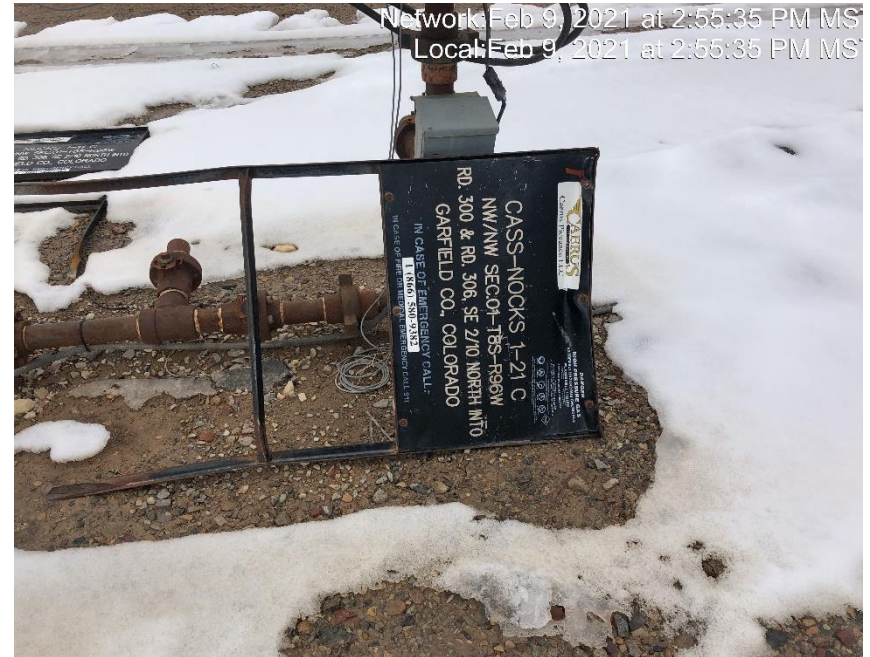
Photo #2865 All wellhead signs missing API number.
