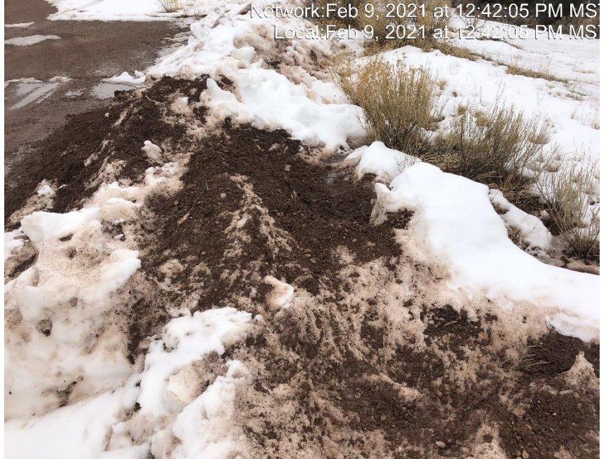
Photo #2857 Sediment has been plowed into berm and vegetation.
