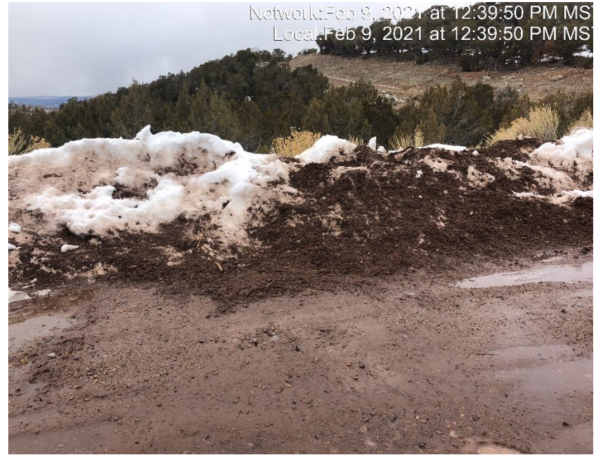
Photo #2855 Sediment has been transported off location due to plowing.
