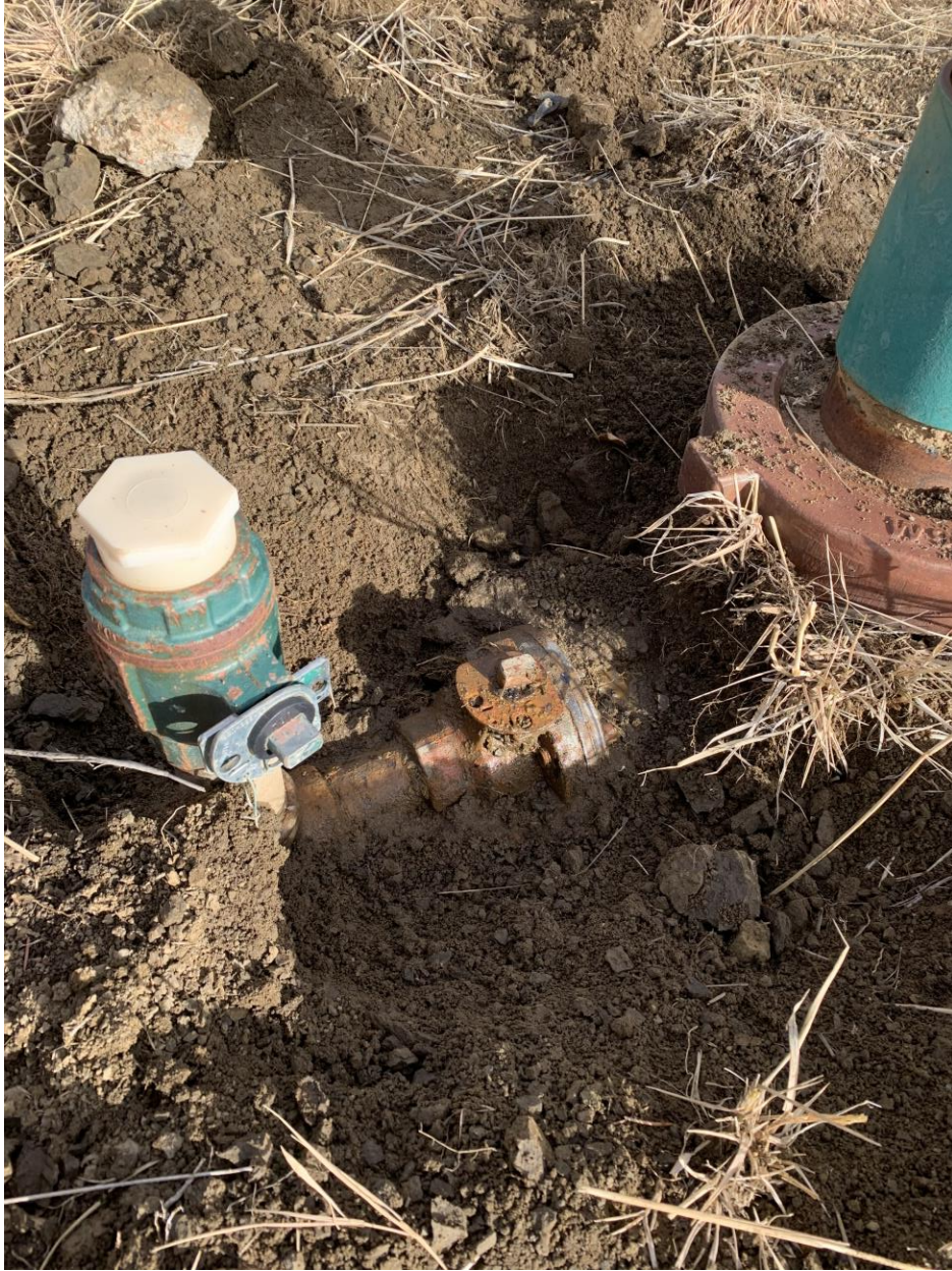
Bradenhead plumped to surface
