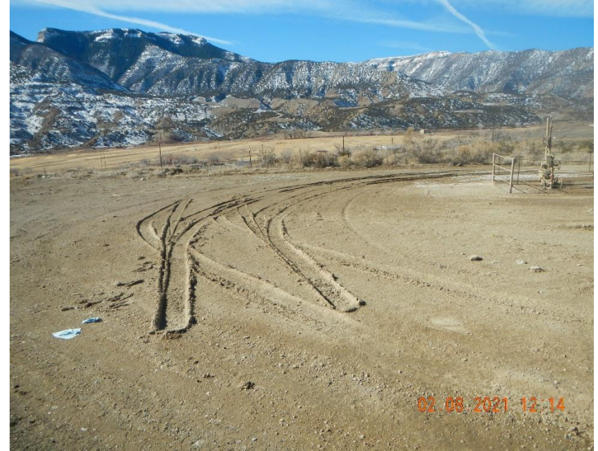
Rutting on location around well head.
