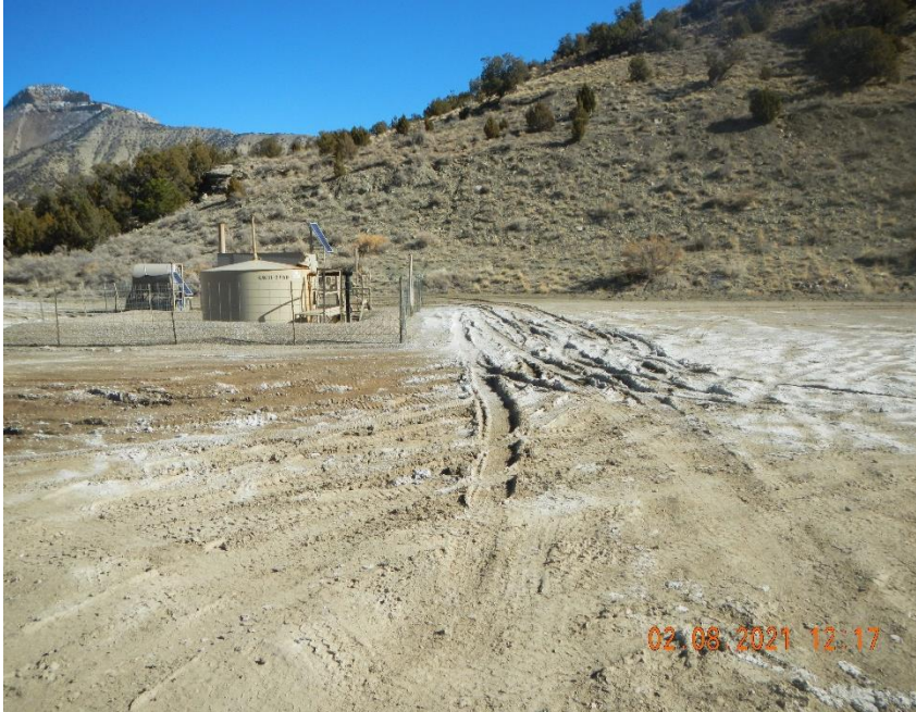
Rutting on location around separator and tank battery.
