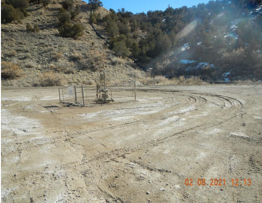
Rutting on location around well head.
