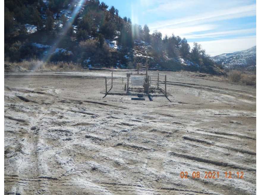
Rutting on location around well head.
