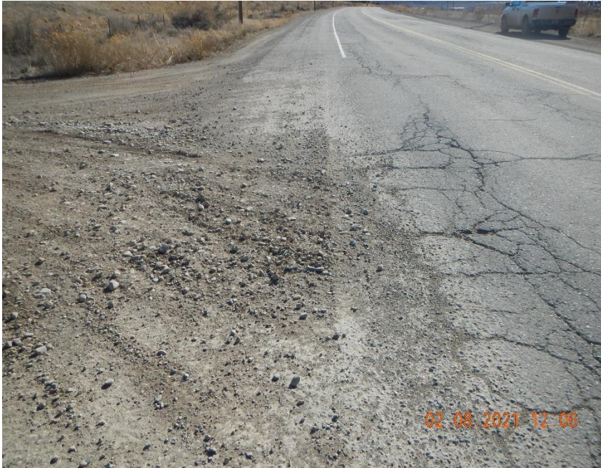
Tracking of sediment at access rd. and CR 215.
