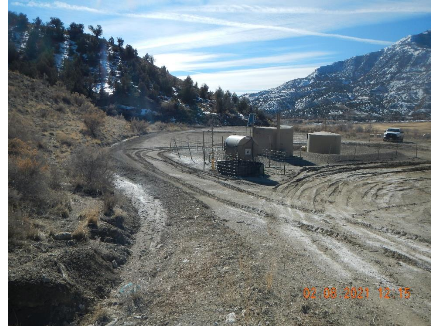
Rutting on location around separator and tank battery.
