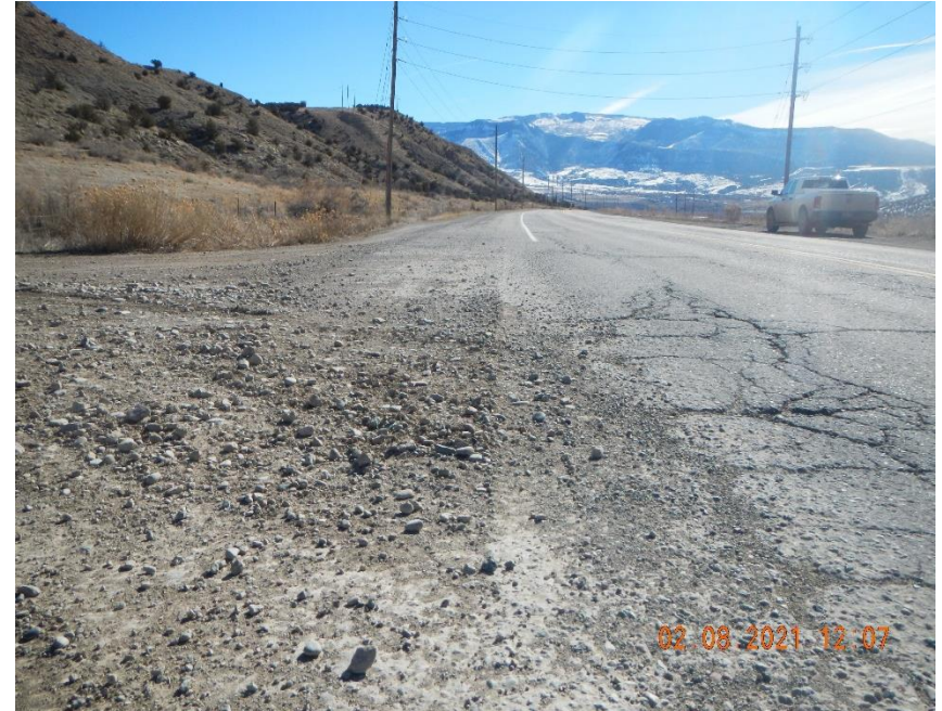
Tracking of sediment at access rd. and CR 215.
