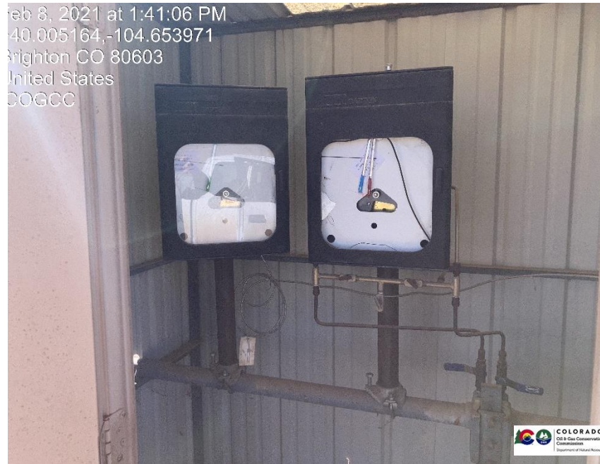
Pic 3 gas meter run with no chart or calibration card
