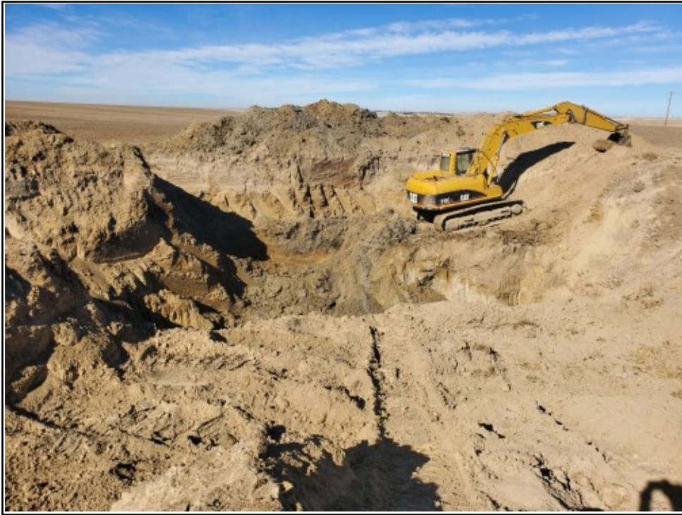
Gulley 1-D Produced Water Pit Excavation – Removal of Gray Pit Bottom Soil
