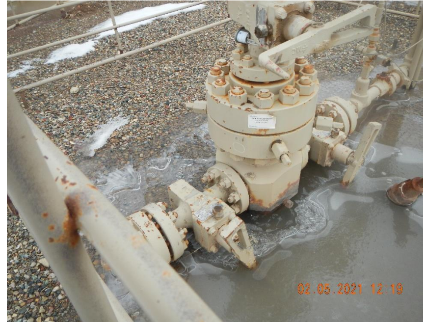
Gas bubbling around surface casing of well.
