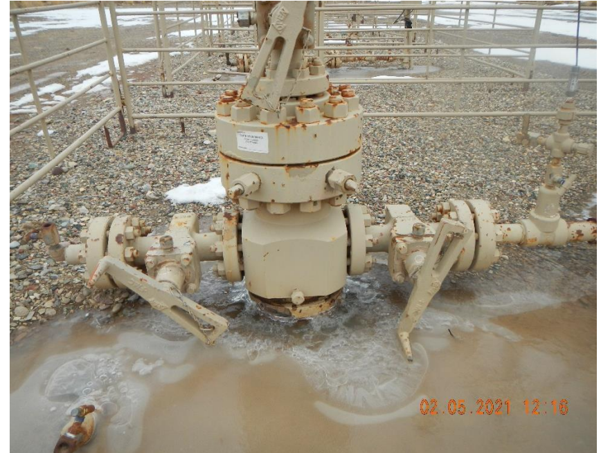
Gas bubbling around surface casing of well.
