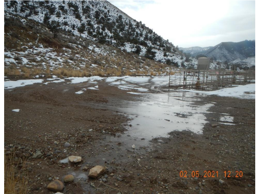
Impoundment of storm water between wells and check dam.
