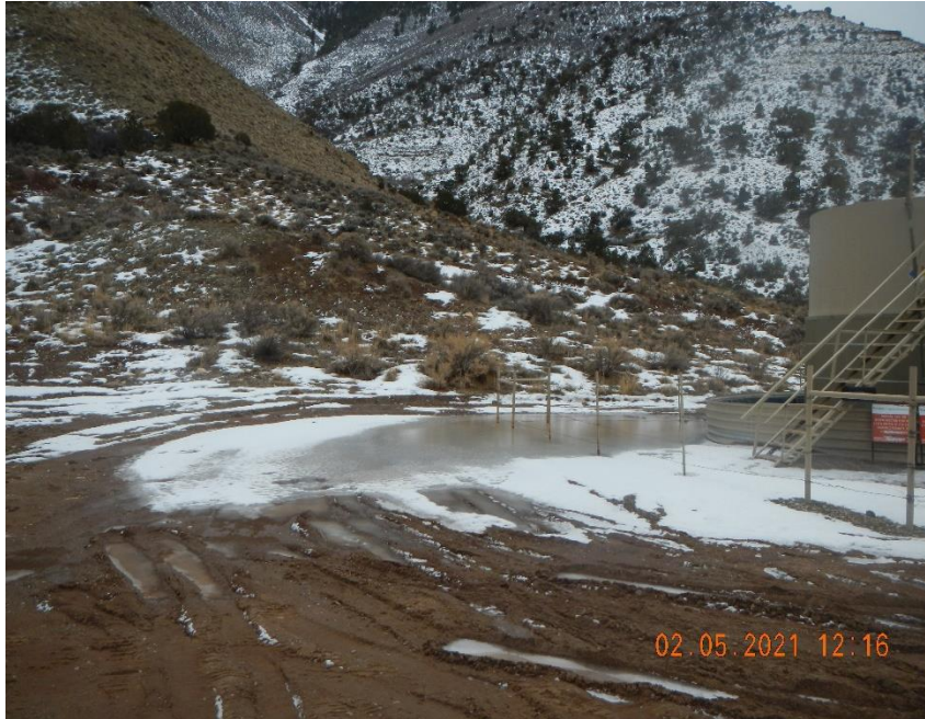
Impoundment of storm water behind tank battery.
