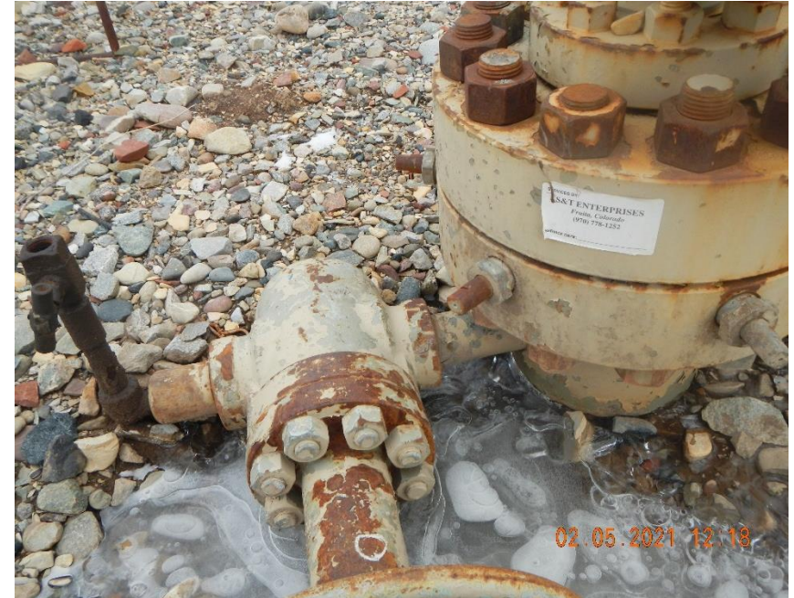
Gas bubbling around surface casing of well.
