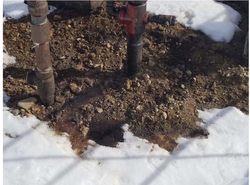
Photo 3. Stained soil at wellhead.
