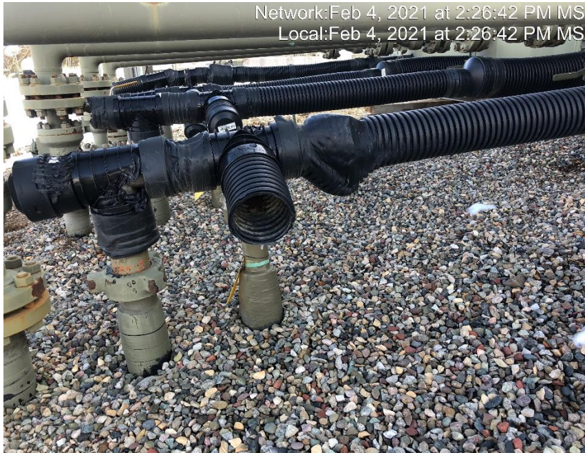
Photo #2819 Flow line exhaust heating insulation open ended and not capped.
