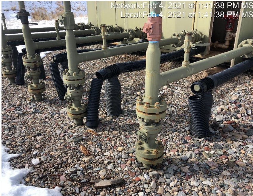
Photo #2812 Multiple flow line exhaust heating insulation open ended and not capped.
