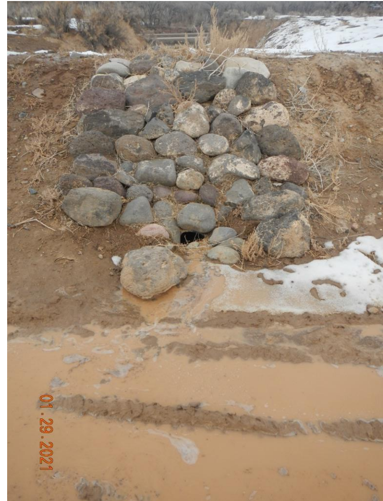
Photo#7: Drains along North berm.
