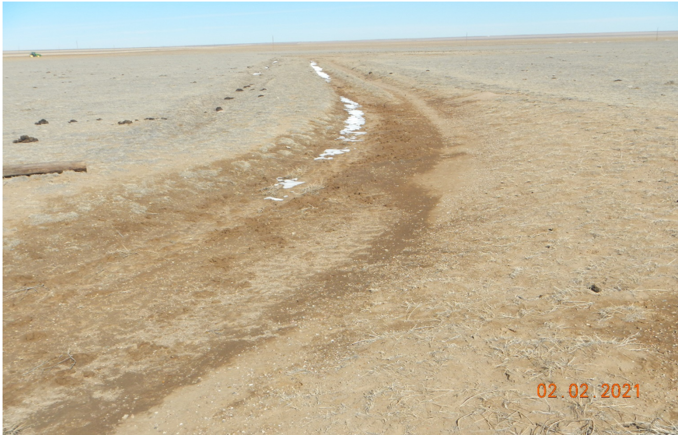
Photo 2. Facing north along the access road associated with the tank battery. The road will need to be recontoured, decompacted, and reclaimed.
