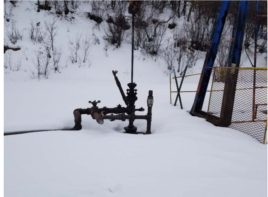
Photo 2. No bradenhead access apparent.
