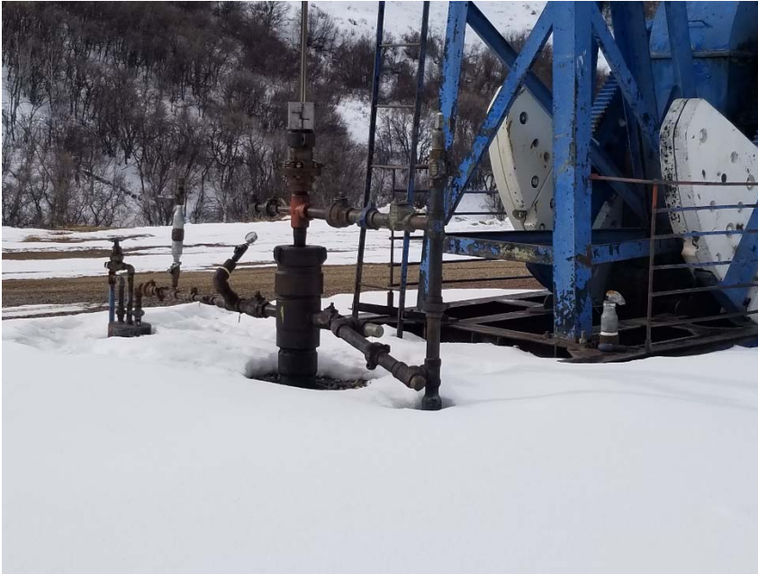
Photo 2. No bradenhead access apparent.
