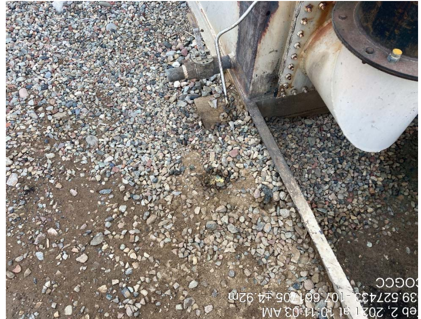
Follow up inspection of staining under stainless blow down (still present)
