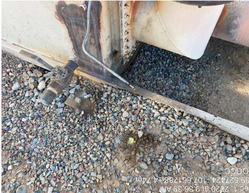
Previous inspection of staining under stainless blow down
