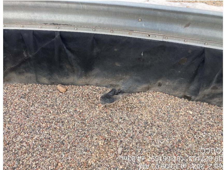
follow up photo of FIXED hole in containment
