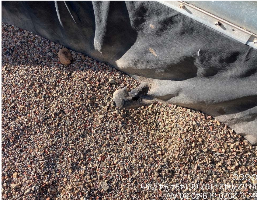
Previous inspection of hole in containment
