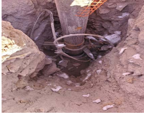
Figure 1: F Wilson #3 Casing Clamps, Hiawatha Field, CO
