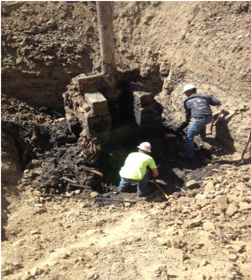
Figure 2: Well Drilled in 1933; Images from Excavation during P&A Operations
