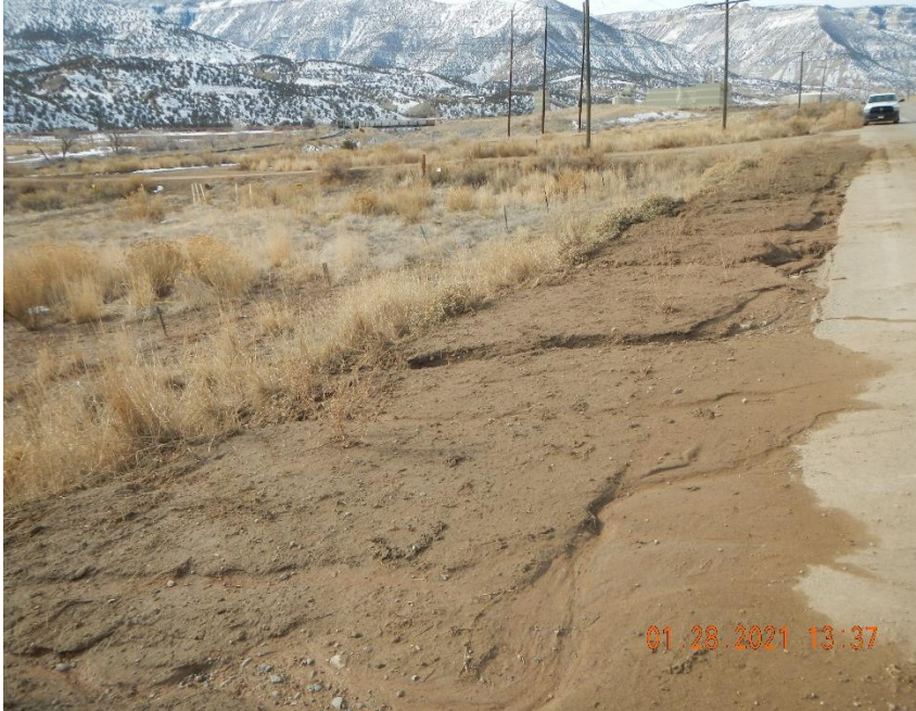
Storm water bmps are failing at access right away and CR215.
