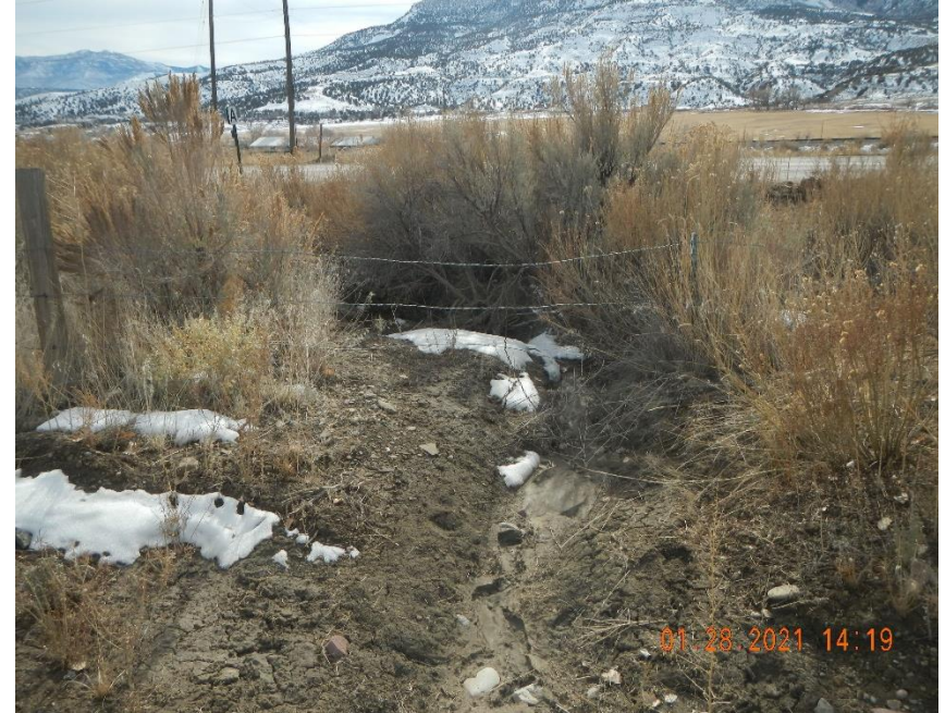
Inadequate ditch for flow.
