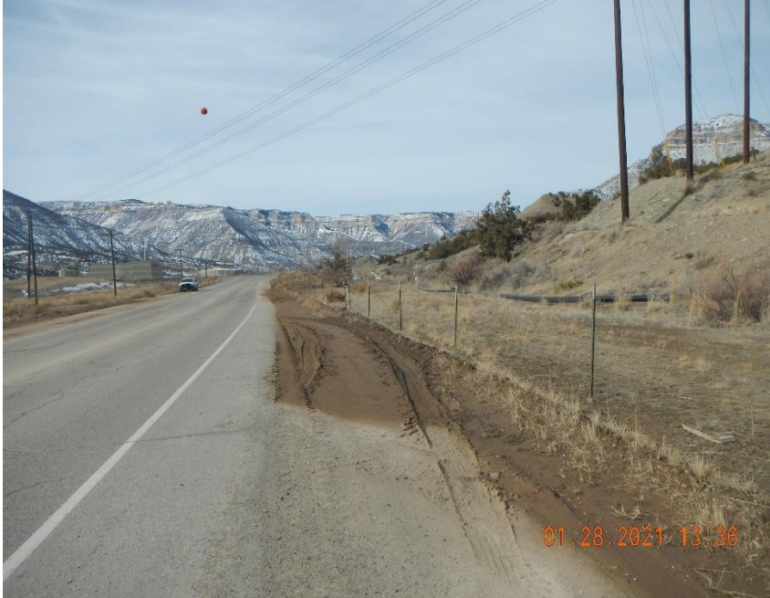
Sediment moving on to shoulder of CR215
