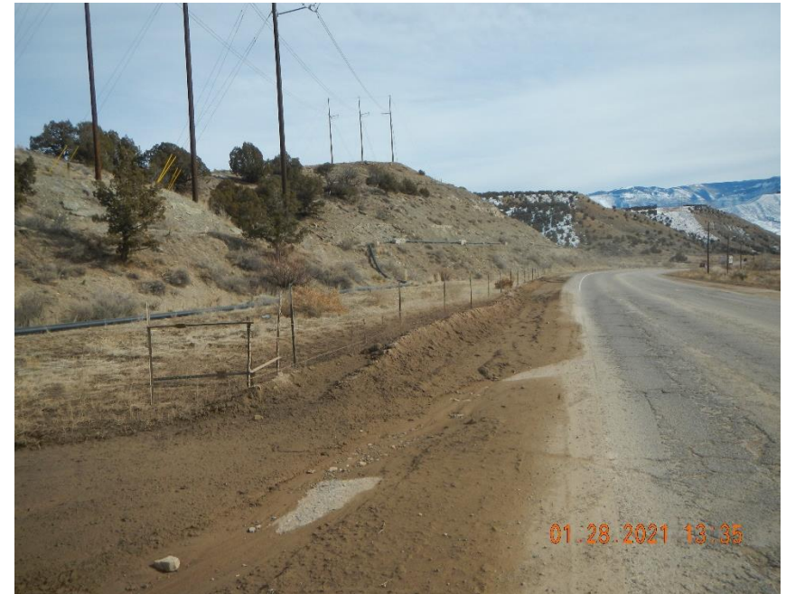
Sediment moving on to shoulder of CR215
