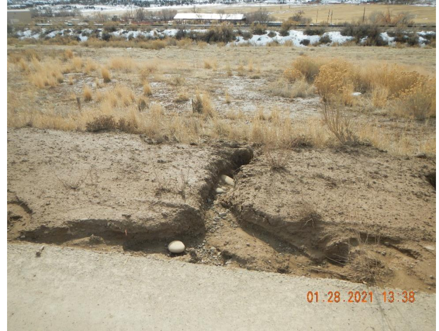
Washing and eroding of shoulder of road.
