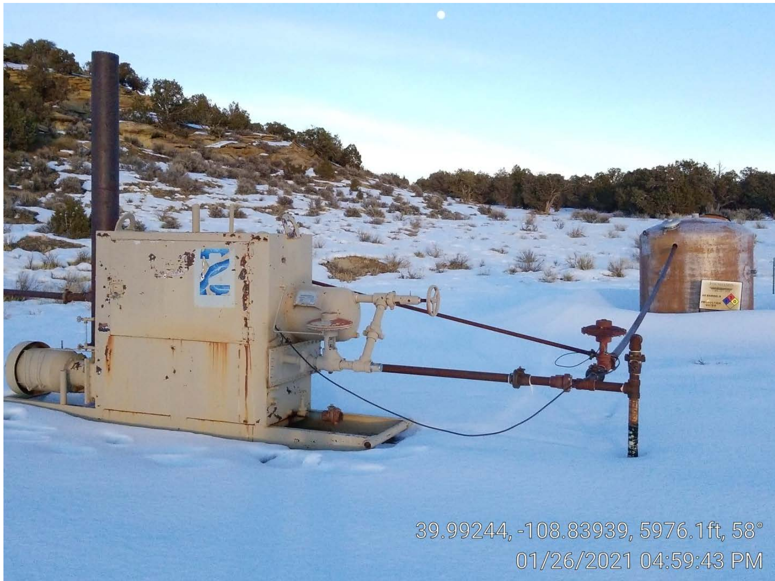
Photo 4. Separator & meter building.
