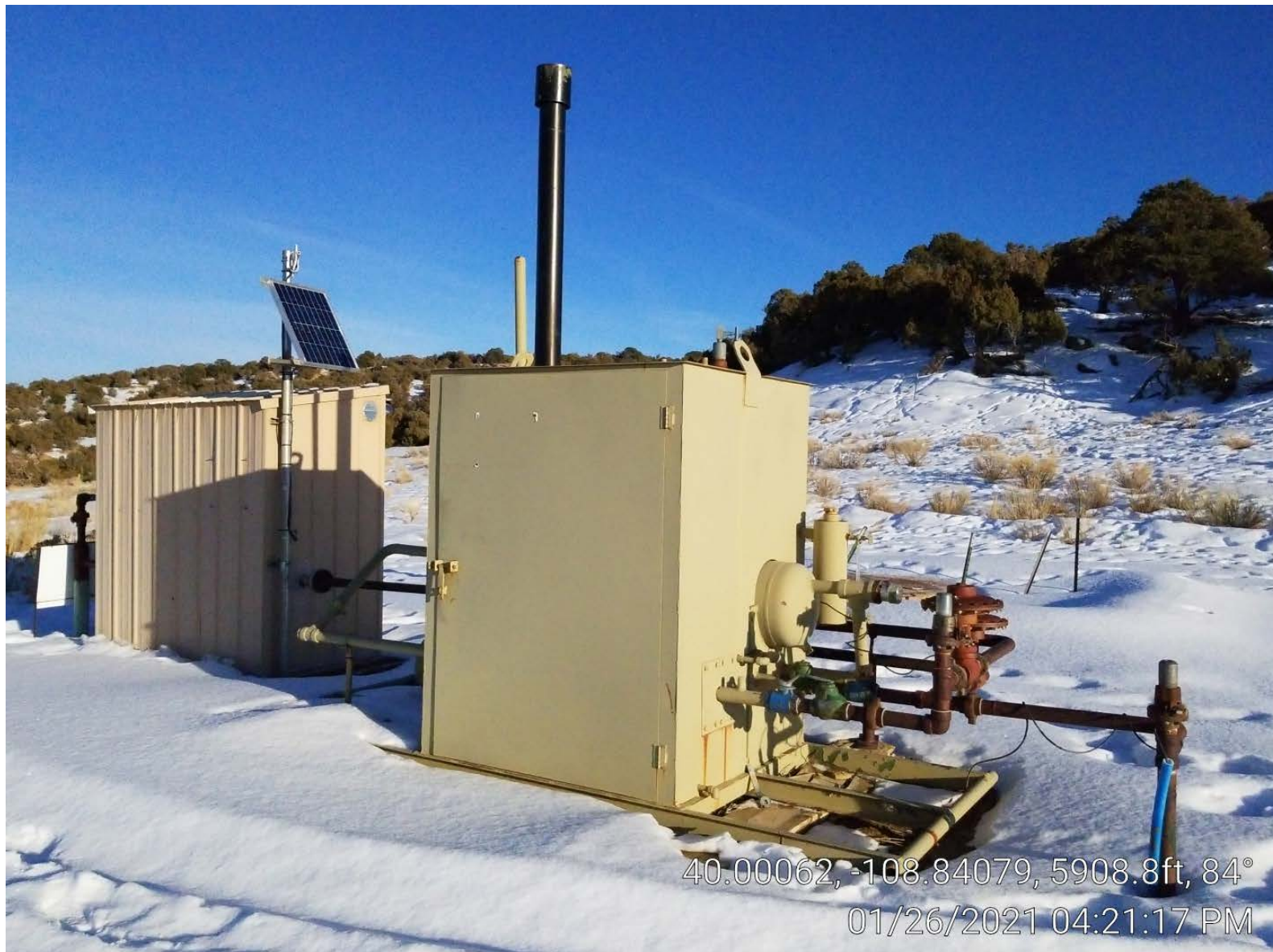
Photo 3. Meter building & separator.
