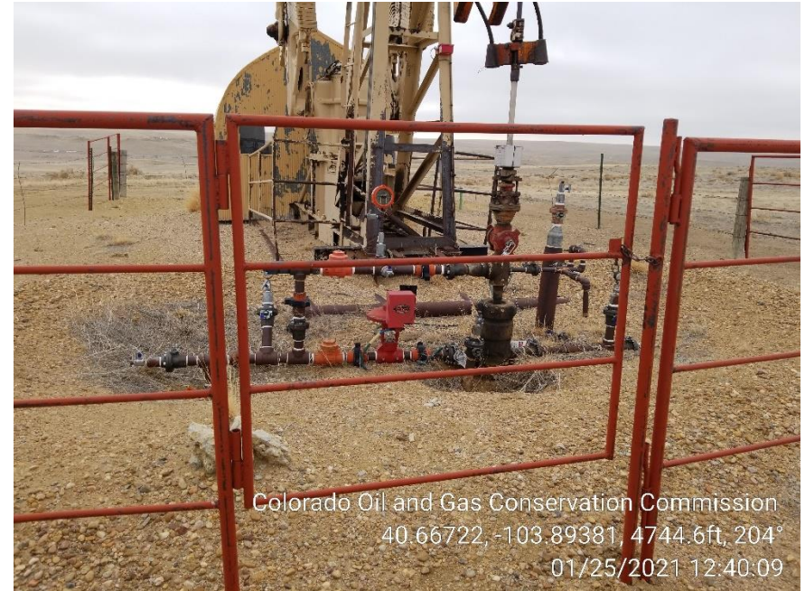
Photo 2 – Wellhead - NO TAG installed
