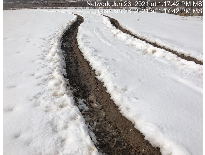
Photo #2716 Ruts present on location due to lack of stabilization.
