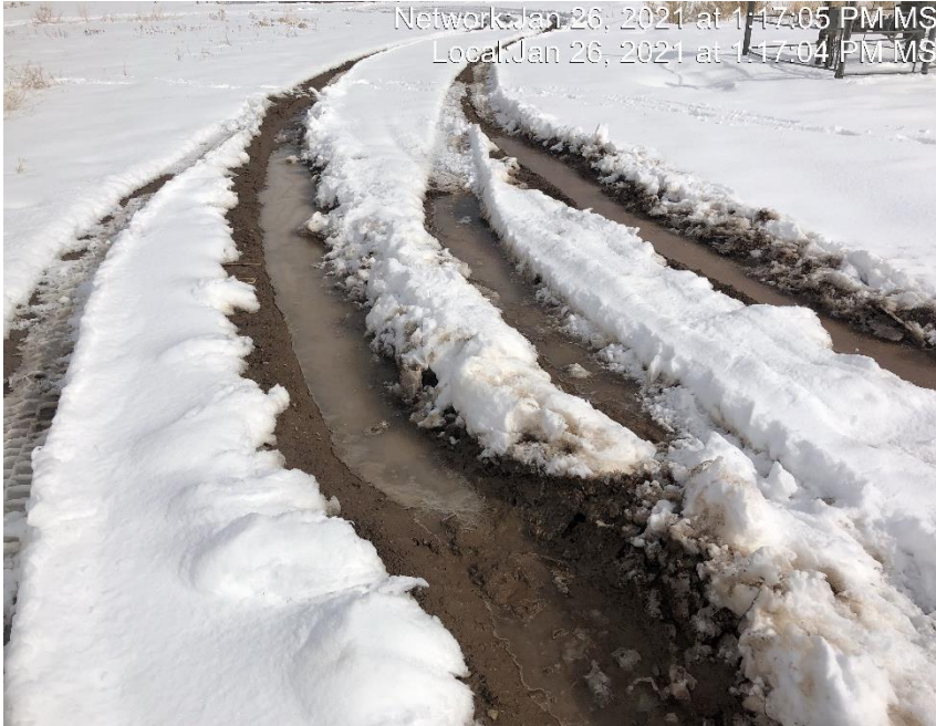
Photo #2715 Ruts present on location due to lack of stabilization.
