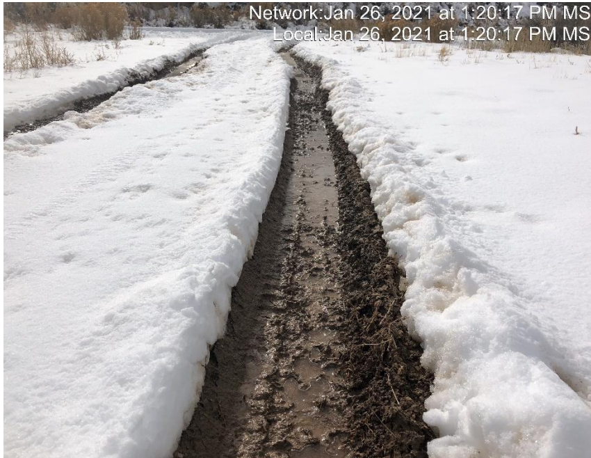
Photo #2717 Ruts present on location due to lack of stabilization.
