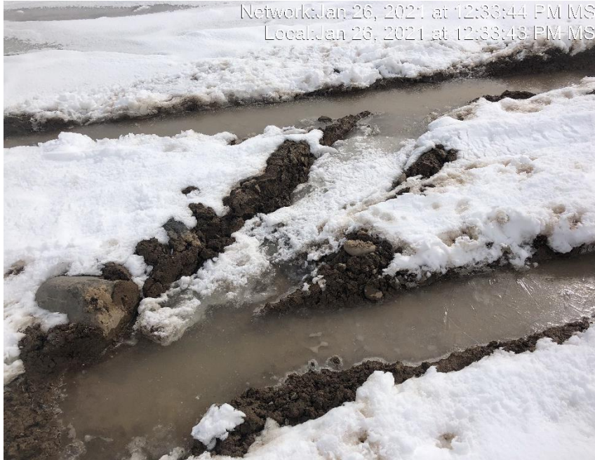
Photo #2708 Rutting present on location due to lack of stabilization.
