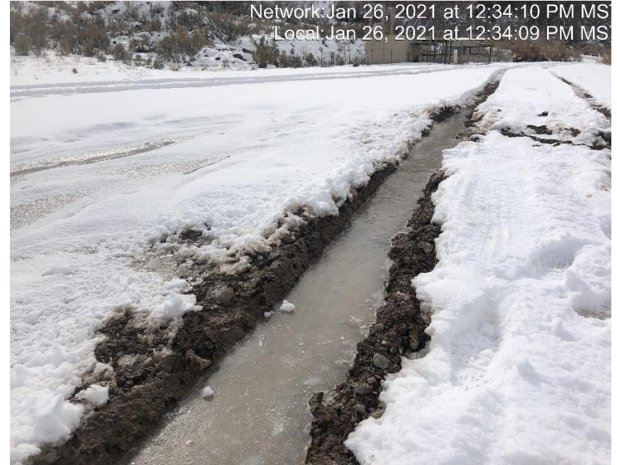
Photo #2709 Rutting present on location due to lack of stabilization.
