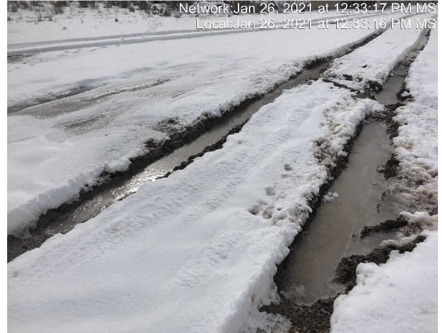
Photo #2707 Rutting present on location due to lack of stabilization.
