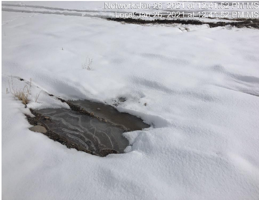
Photo #2710 Rutting present on location due to lack of stabilization.
