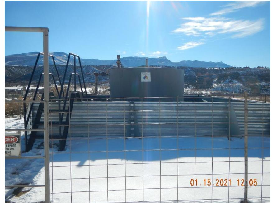
**Capacity on Produced water tank is less than the size of the lettering size on label and can not be seen from distance of 100'.**
