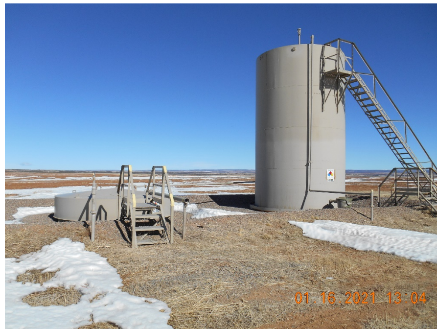
Tank Battery with earth berms.
