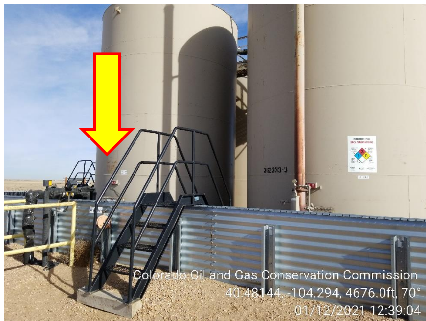
Photo 3 – NW Tank (Water Tank) missing NFPA
