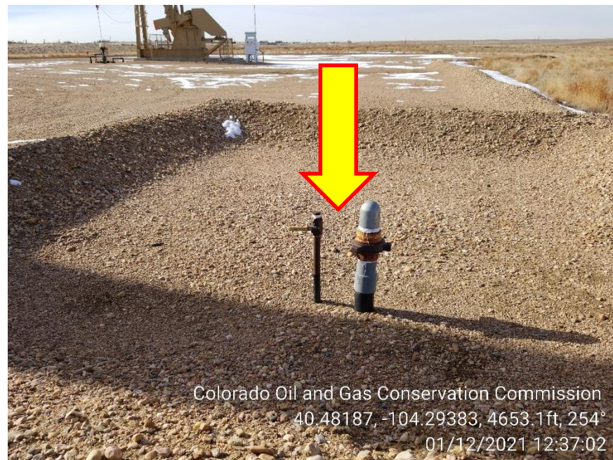
Photo 6 – Unmarked Risers in the NE Corner
