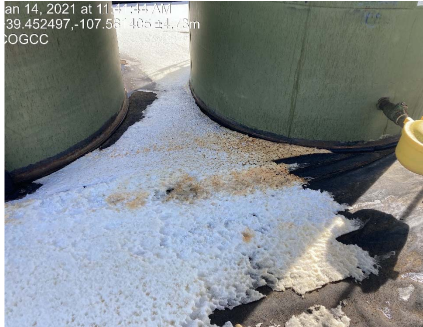
Staining from tanks/blowing down high pressure line
